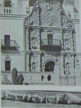
Left: Time and the elements were taking their toll before restoration. Note missing columns. Right, top The facade now, Below: Units of a cast column before installation.
